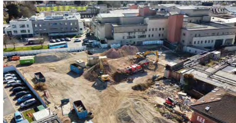
Aerial view of the Dyson Cancer Centre site
