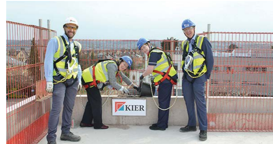
The Dyson Cancer Centre construction, including the all-important Topping Out ceremony
