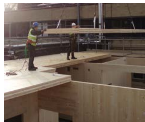
New NICU construction begins
